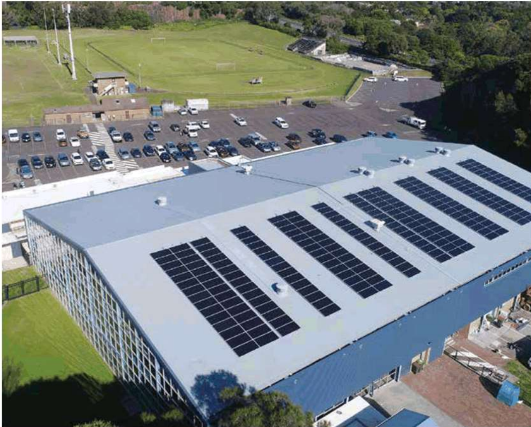
Kiama Leisure Centre - 99.6kW Photovoltaic system.
