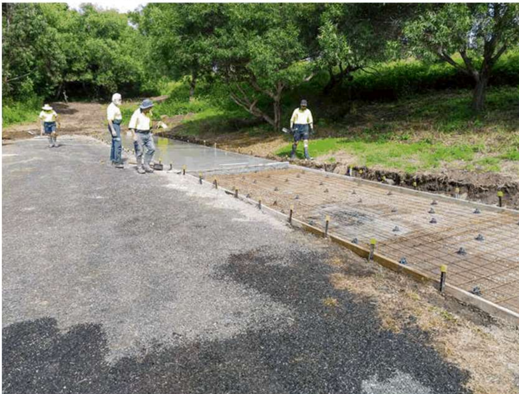
BMX Track Construction commences at Sanctuary Place
