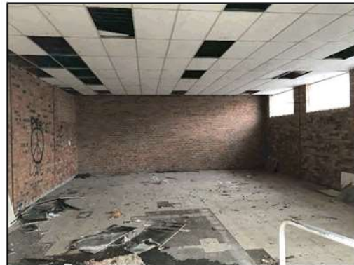
Figure 27. View to the interiors of the former hardware store as viewed from within the building, facing south. Note the broken suspended ceilings and tiled flooring.
