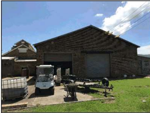
Figure 16. External view to the rear of Shed as viewed from within the site, facing west. Note the later addition metal roller doors.
