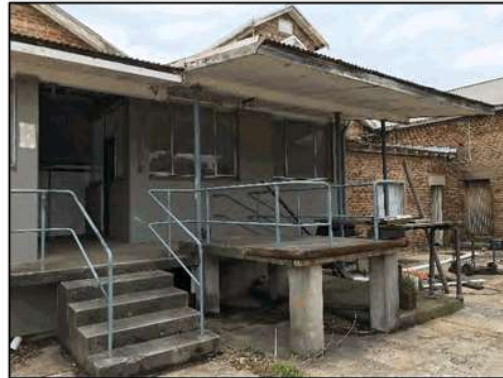
Figure 19. View to the later addition kitchen and the office located to the rear of Milk room 1 and 2 as viewed from within the site, facing west. Note the non-original fabric of the kitchen and office including the later addition concrete platform.
