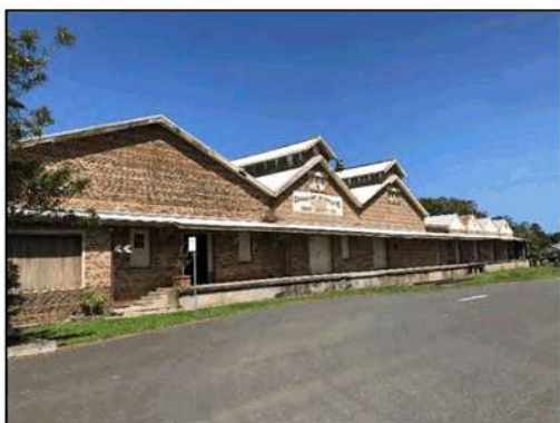
Figure 12. View to the former Gerringong Dairy Co-Op as viewed from the carparking of Gerringong station, facing south-east.
