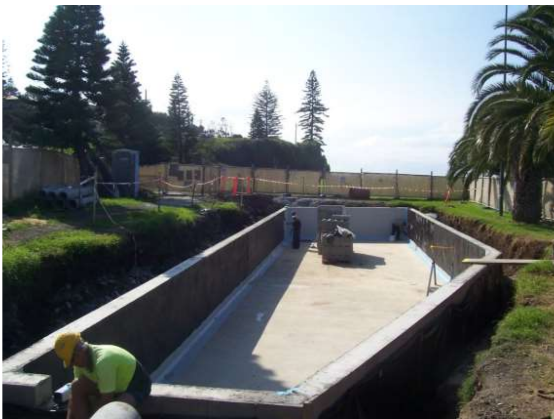
Figure 3 – construction of underground tank at Black Beach
