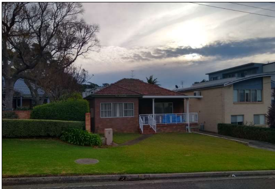
Figure 2 – Site Photograph (View of Existing Dwelling to be demolished)
