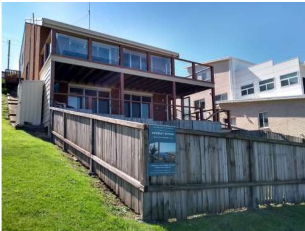
Figure 7 – Site photograph of existing dwelling from the south-west
