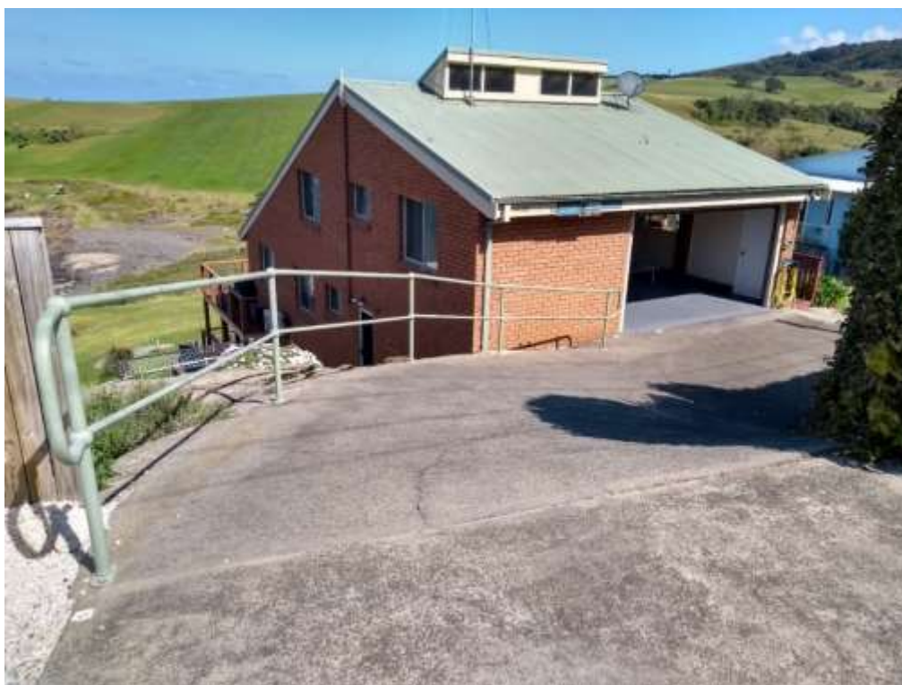
Figure 5 – Site photograph of existing dwelling from north-east
