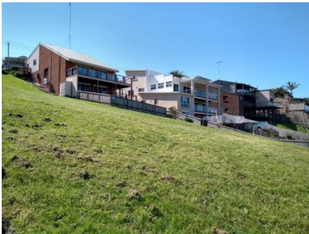
Figure 10 – Site photograph of existing dwelling from the south-west
