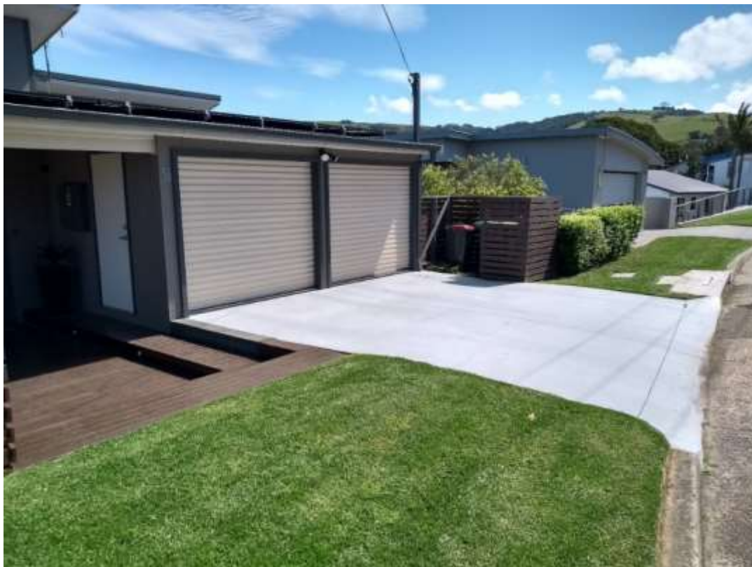
Figure 23 – Site photo of 36 Anembo Crescent, Kiama Heights
