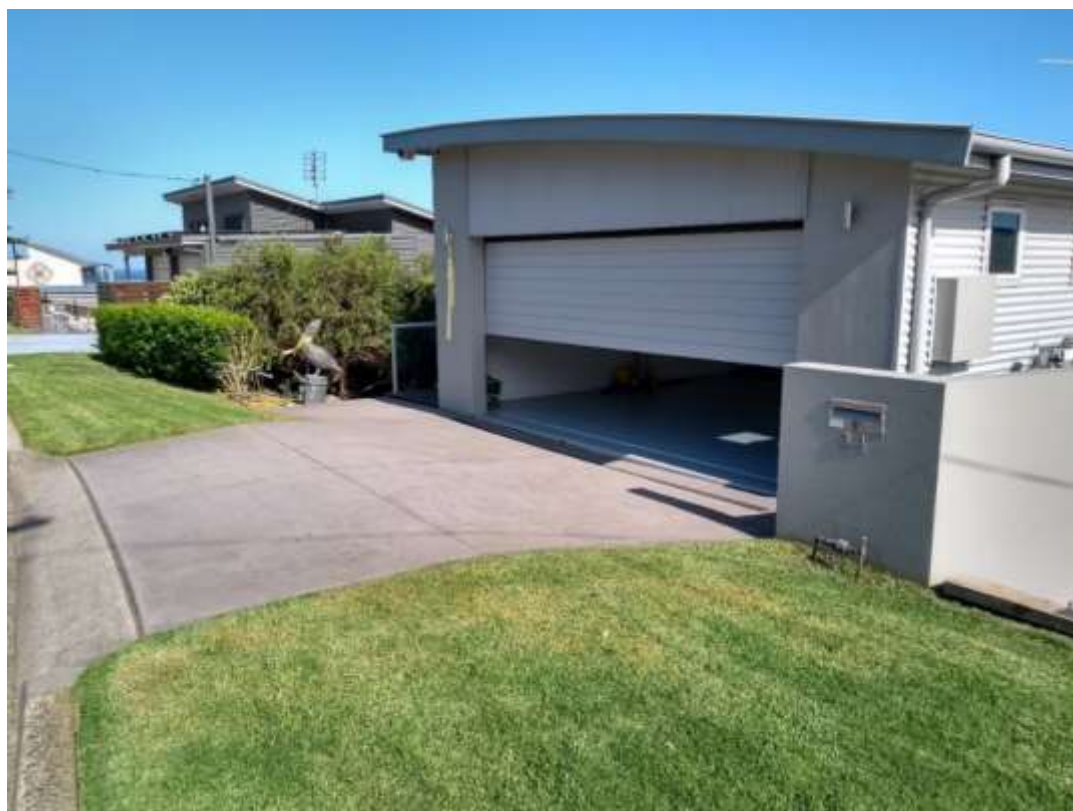
Figure 24 – Site photo taken at 34 Anembo Crescent, Kiama Heights
