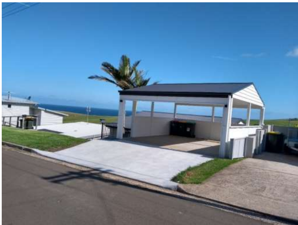
Figure 25 – Site photo taken at 30 Anembo Crescent, Kiama Heights
