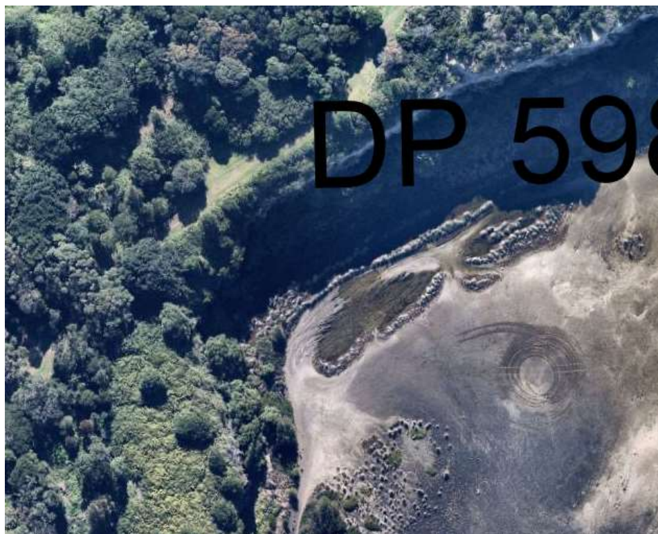
Figure 3 – Development site photograph (2019/20 View, ↑N)
