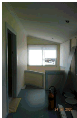
Figure 4.48 View north of the enclosed rear verandah showing staircase to the basement.
