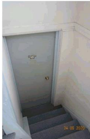
Figure 4.50 Detail of the entrance to the basement.
