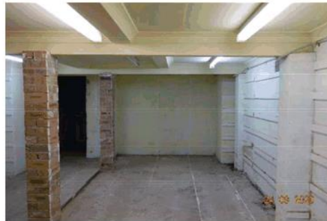
Figure 4.52 Basement (looking west) showing detail of exposed brick supports.
