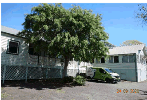
Figure 4.17 View of the rear parking area in the northeastern corner of the site, looking towards the eastern elevation of the house.
