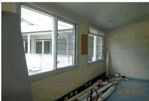
Figure 4.47 View of the enclosed southern verandah showing the contemporary louvered windows and lino flooring.
