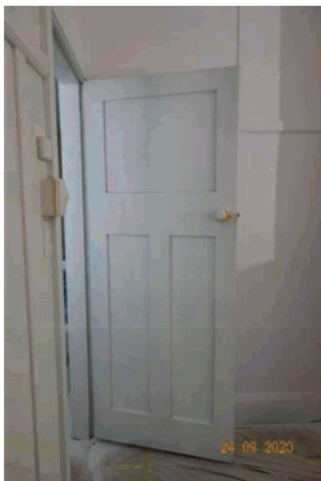
Figure 4.27 Original timber door with contemporary hardware in the southwestern room.
