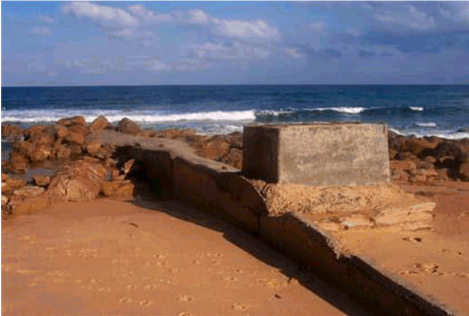
Photo - Outlet of old drainage structure
