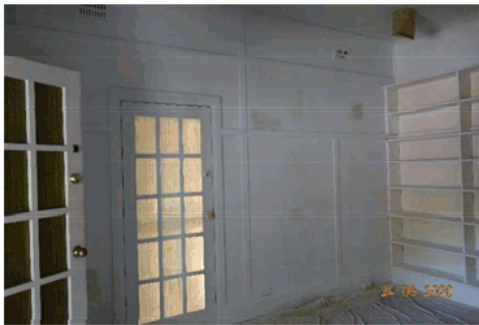
Figure 4.21 Entrance foyer (looking northeast) showing the contemporary joinery.
