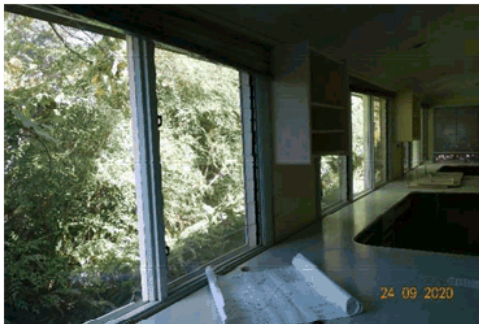
Figure 4.33 Detail of inset desks in enclosed verandah and new sliding windows facing southwest.
