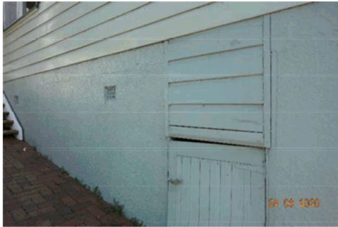
Figure 4.19 Detail of the entry to the basement area.
