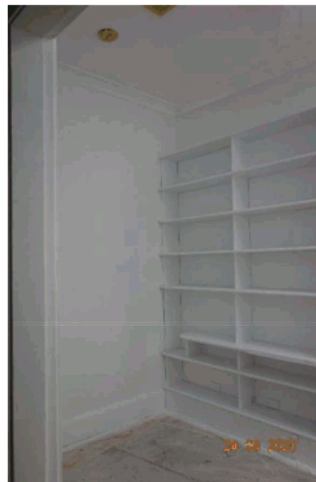
Figure 4.44 Detail of the contemporary joinery.
