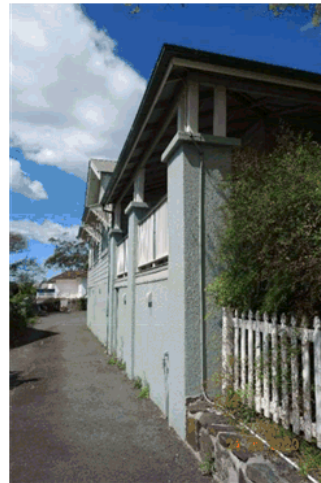
Figure 4.14 View of the northern elevation from driveway showing the elevated foundations.
