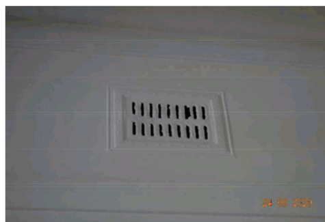
Figure 4.24 Original wall vent in entrance foyer.
