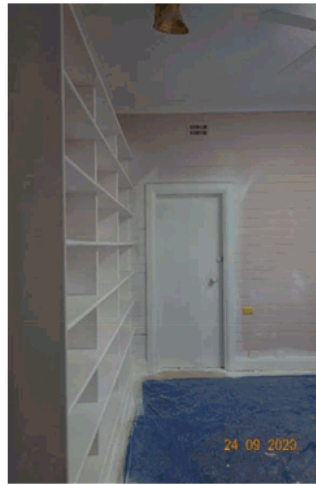
Figure 4.62 View of a rear room in the weatherboard extension showing timber-panel walls with contemporary joinery and door.
