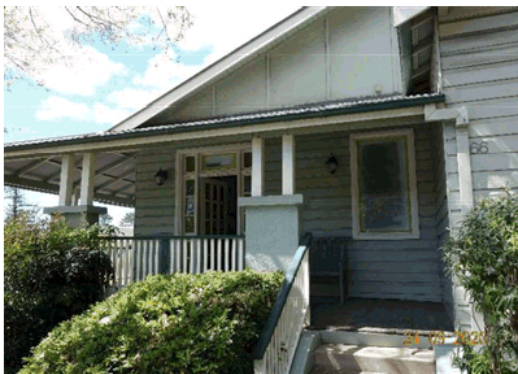
Figure 4.10 Detail of west elevation showing the open verandah with contemporary timber balustrade.
