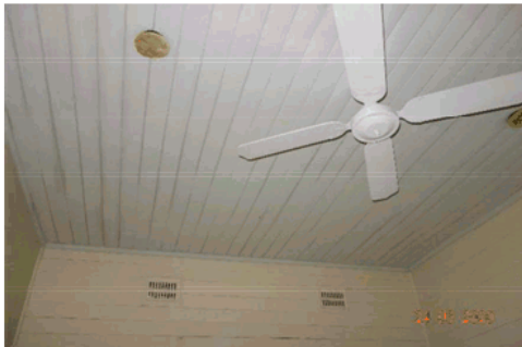
Figure 4.59 Detail of ceiling, fan and vents in kitchen.
