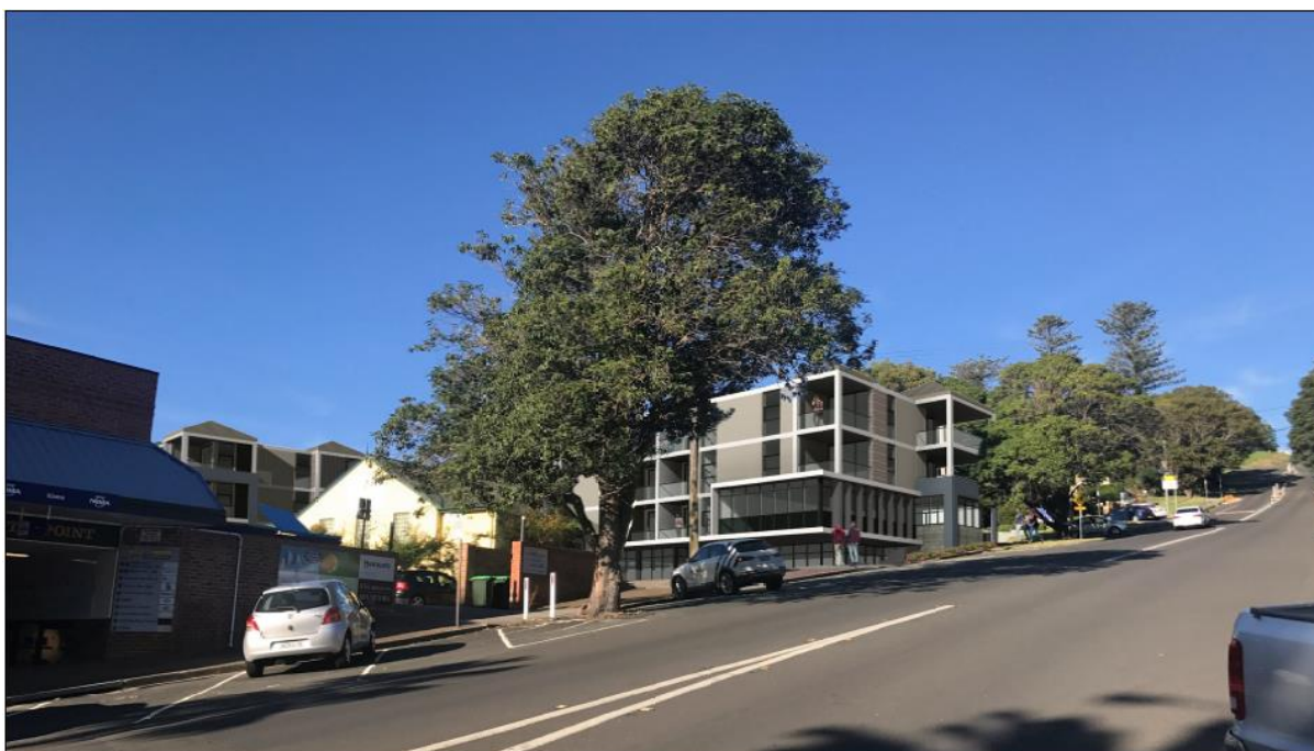
Figure 1 – Looking south along Collins Street
