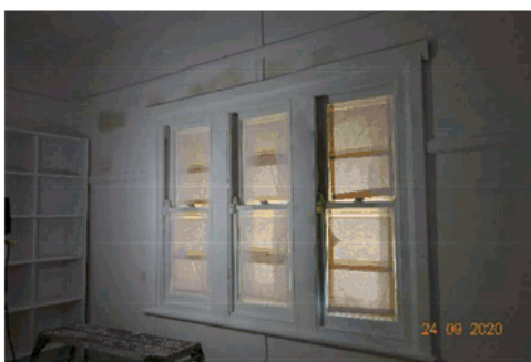
Figure 4.29 Original double-hung windows that face west onto Collins Street.
