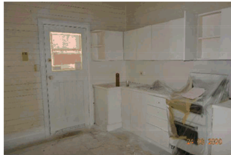
Figure 4.60 View of the kitchen showing fittings.
