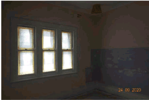
Figure 4.41 View of a northern room with painted skirting and contemporary cornices looking towards the window.
