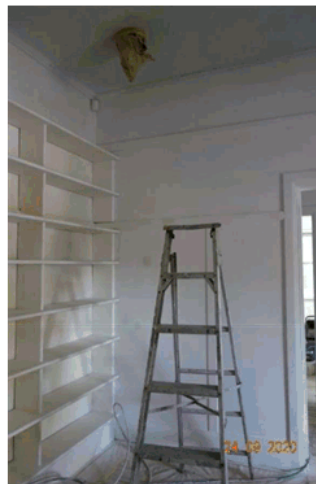
Figure 4.22 Entrance foyer (looking south) showing timber details on the wall and original skirting.
