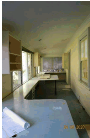
Figure 4.32 Enclosed verandah (facing west) showing the original timber-framed windows to the north that were formerly external.
