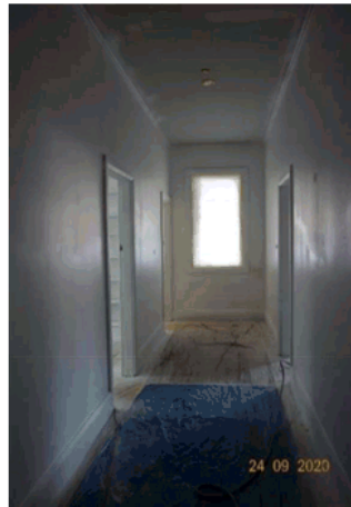
Figure 4.36 View of the central corridor facing west.
