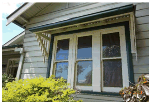
Figure 4.12 Detail of the timber-framed window on the gable bay with contemporary awning.
