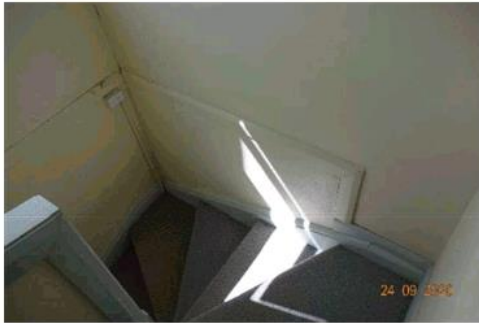
Figure 4.49 Detail of the carpeted stairs that lead to basement.
