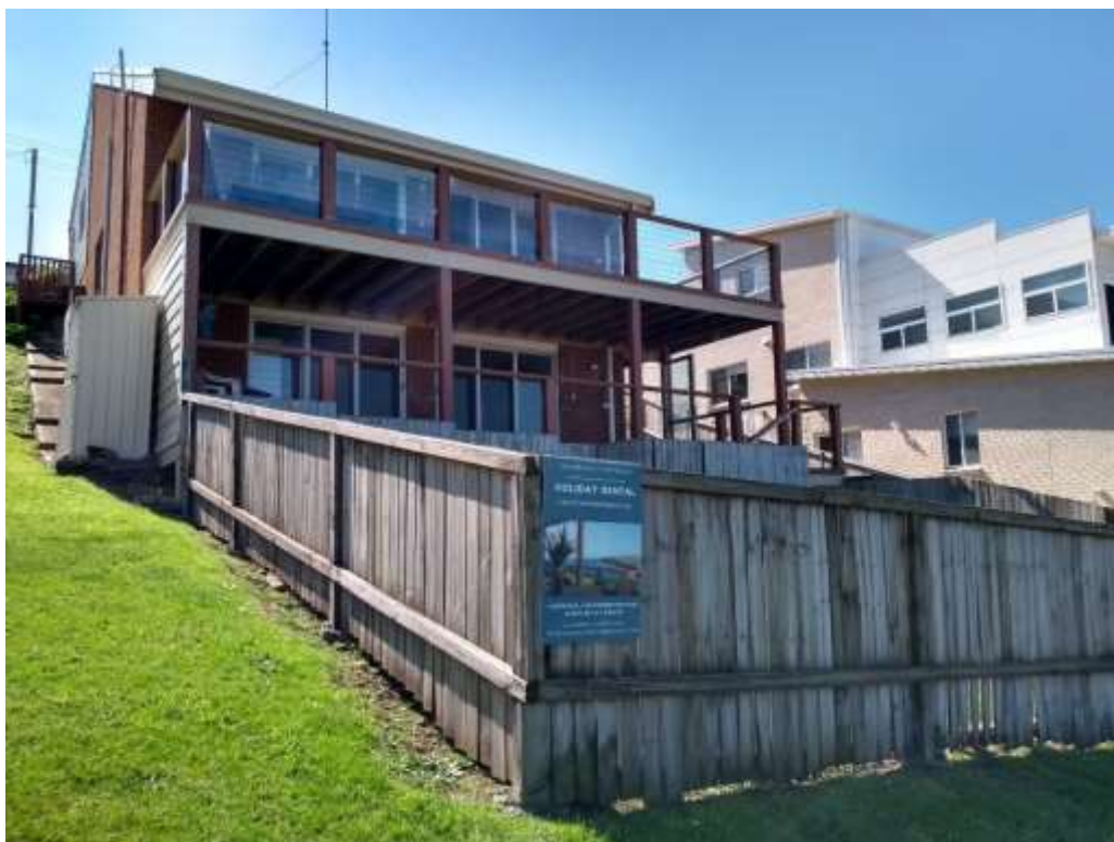
Figure 6 – Site Photograph of existing dwelling from southwest
