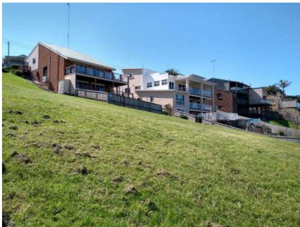
Figure 9 – Site Photograph of existing dwelling from southwest
