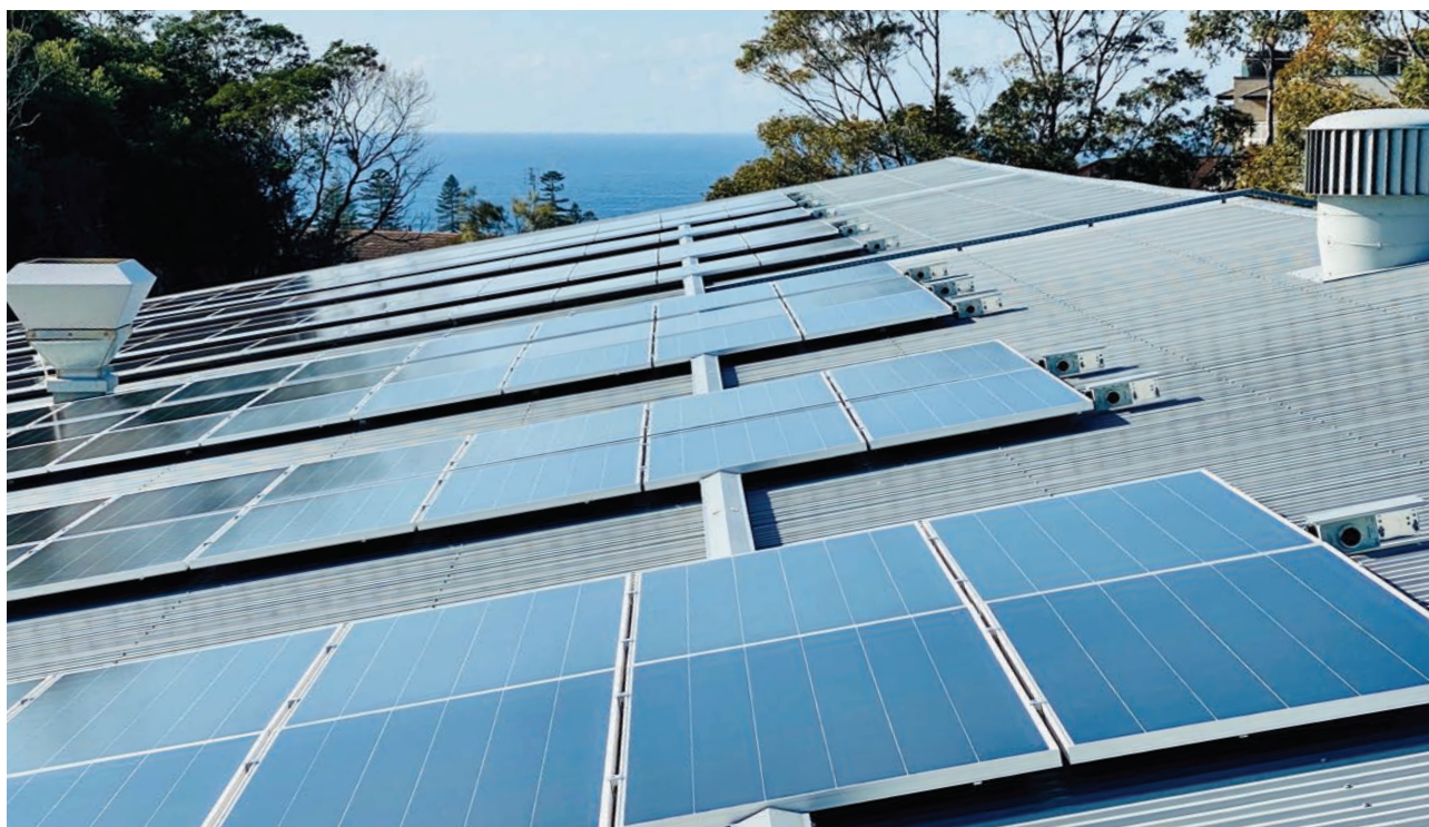
Kiama Leisure Centre - 99.6kW Photovoltaic system reduces energy consumption on site by 30% annually.
