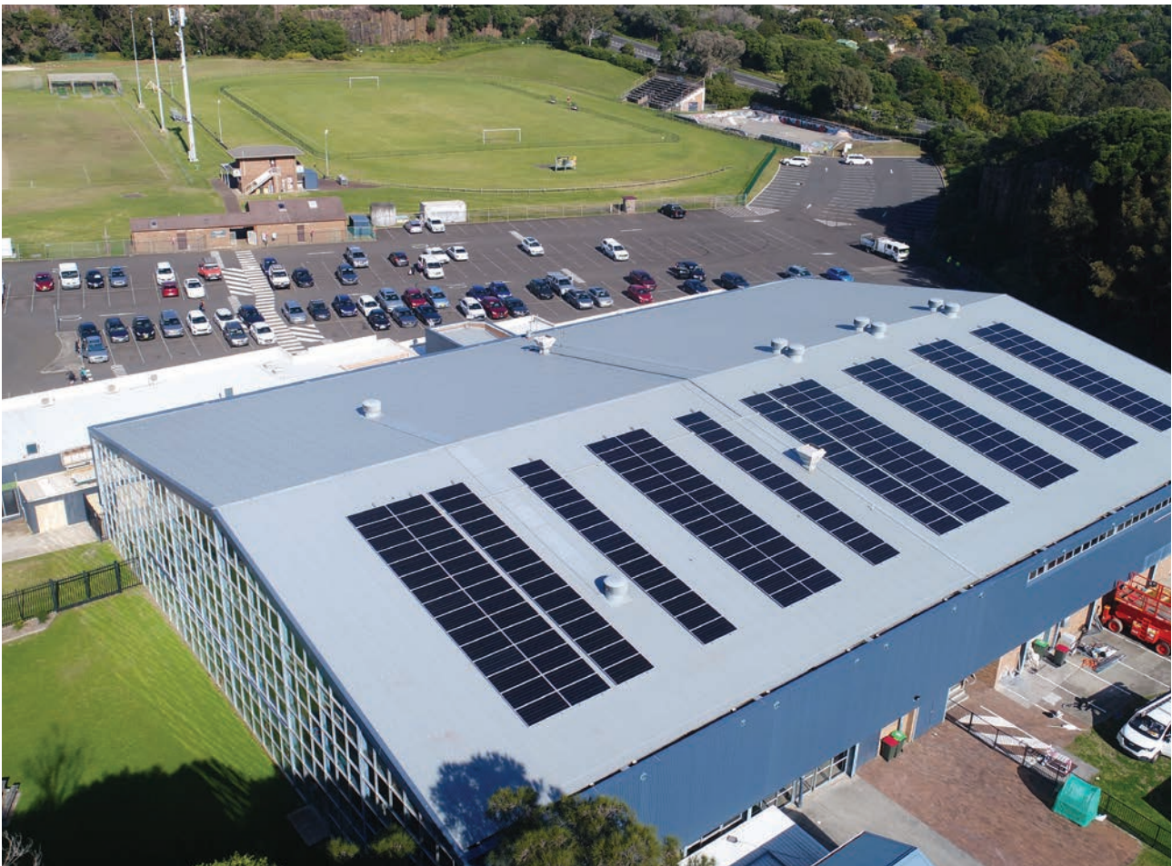
Kiama Leisure Centre - 99.6kW Photovoltaic system.
