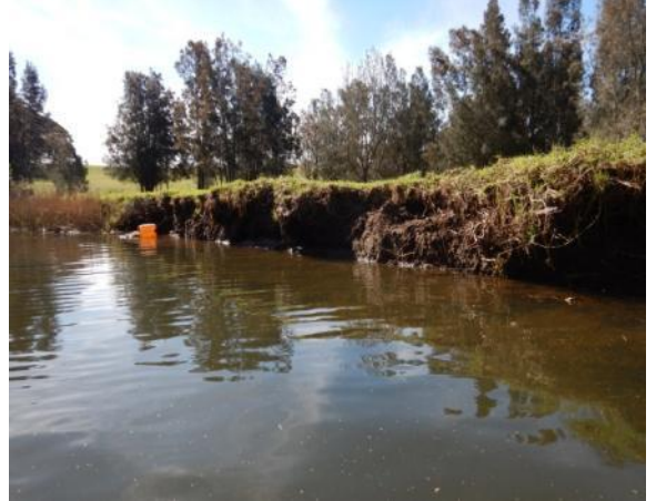
Site 14 – Downstream Swamp Road (D. Wiecek, 2014)
