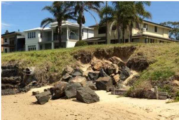
Site 5 – Charles Avenue foreshore (this site has been repaired)
