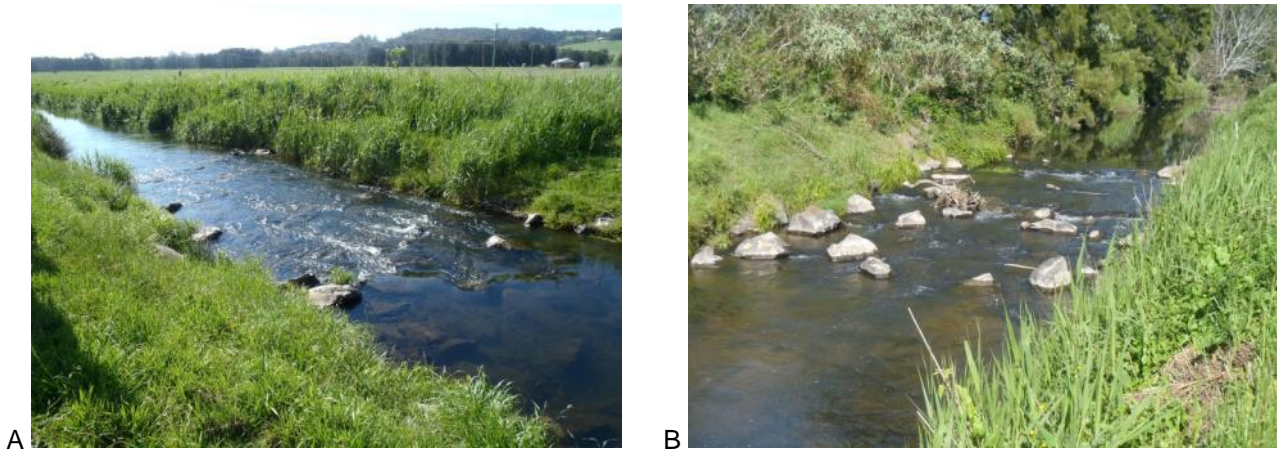
Figure 32: Terragong Drain rock ramps
