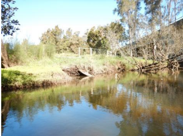
Princes Highway bridge (D. Wiecek, 2014)
