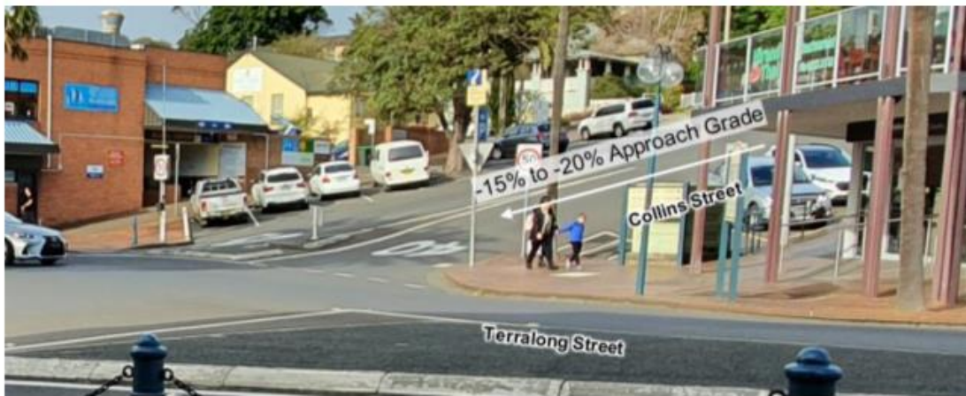
Figure 9.6: Collins Street Southern Approach Gradient to Roundabout
