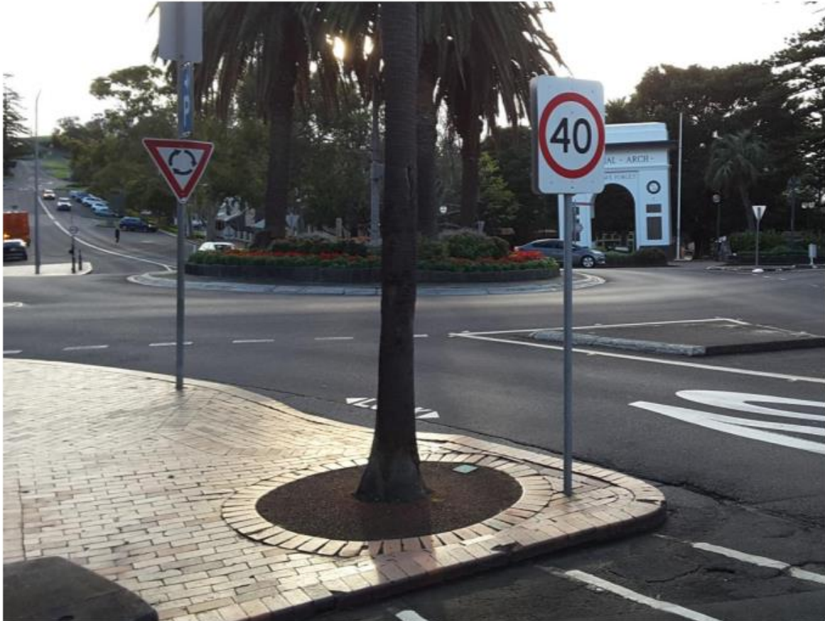
Figure 9.5: Sight Line Issues due to Roundabout Vegetation
