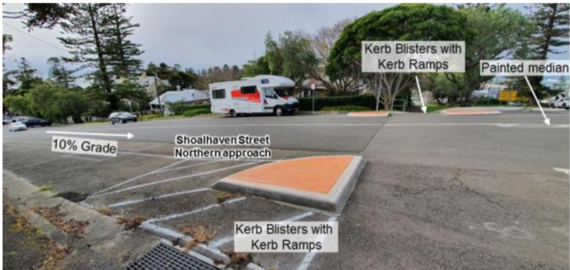
Figure 9.17: Bong Bong Street/Shoalhaven Street Existing Conditions (Shoalhaven Street Northern Approach)
