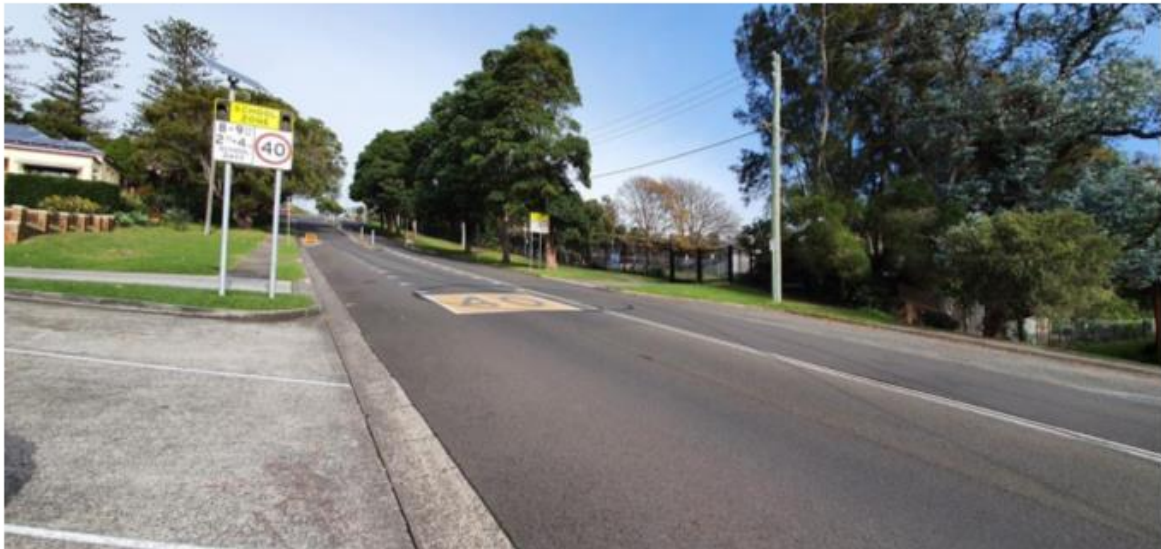
Figure 9.10: Collins Street Steep Down Hill Approach to the Proposed Crossing
