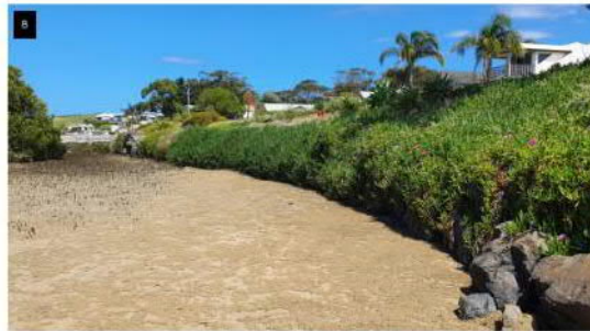
8. Well vegetated rock wall in excellent condition due to protection offered by mangroves.
