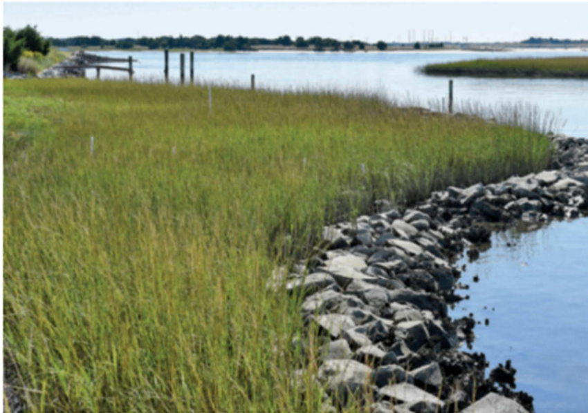
Figure 5-7 Examples of Riprap Shoreline Protection
