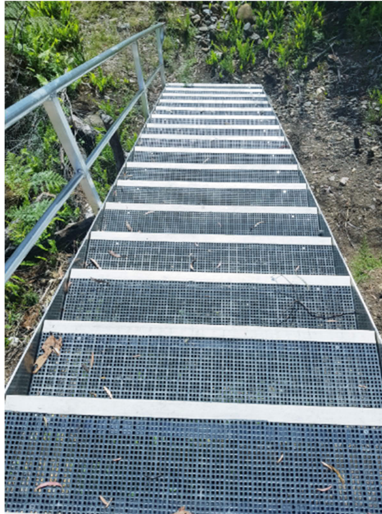
Figure 5-19 Example of FRP Mesh Beach Access Steps as an Alternative to Concrete
