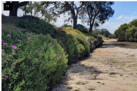
11. Vegetated rock wall in excellent condition. Consider adding scour protection along toe.
