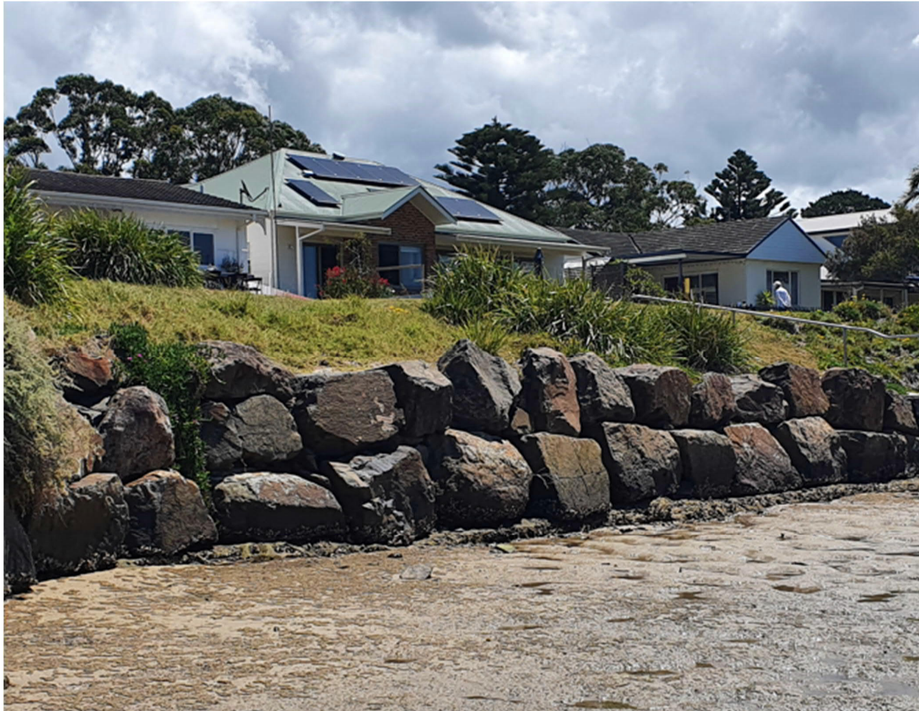
Figure 5-17 Example of Existing Rock Wall Treatment (Note no scour protection shown– to be incorporated)
