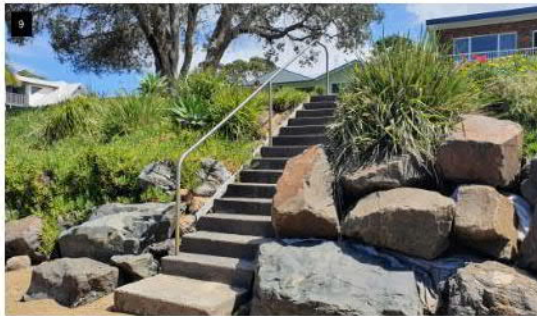
9. Concrete stairs in good condition. Add rock scour protection around base of stairs or piles.
