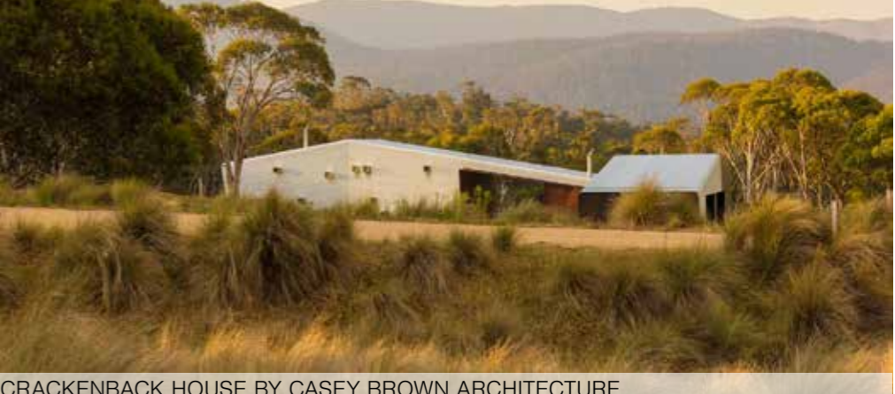
CRACKENBACK HOUSE BY CASEY BROWN ARCHITECTURE
