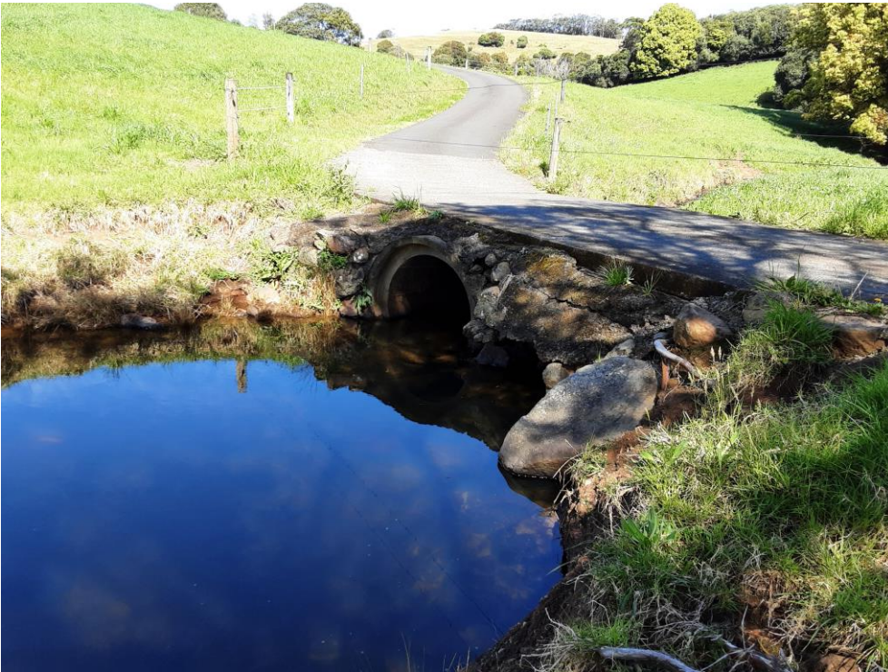
Photo 18 Disturbance associated with bridge construction and paved access roads
