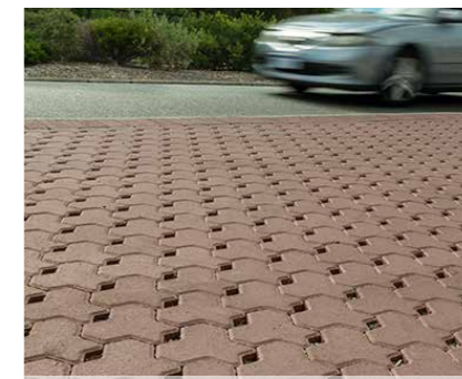
Permeable parking bays
